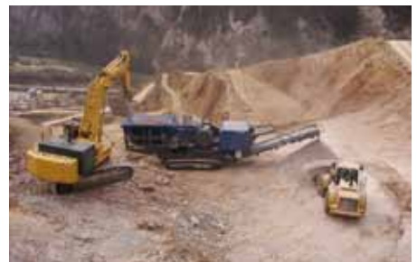
Crushing of hard stone in Austria.
