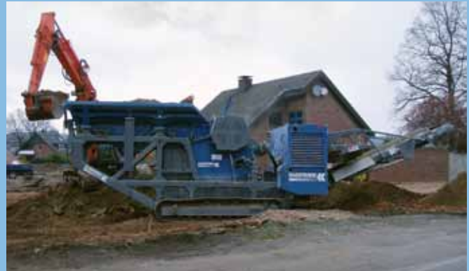
MC 100 R processing demolition waste.
