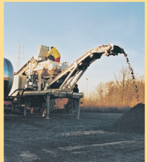
Mobile cold recycling mixing plant producing cold-mix materials with foamed bitumen.
