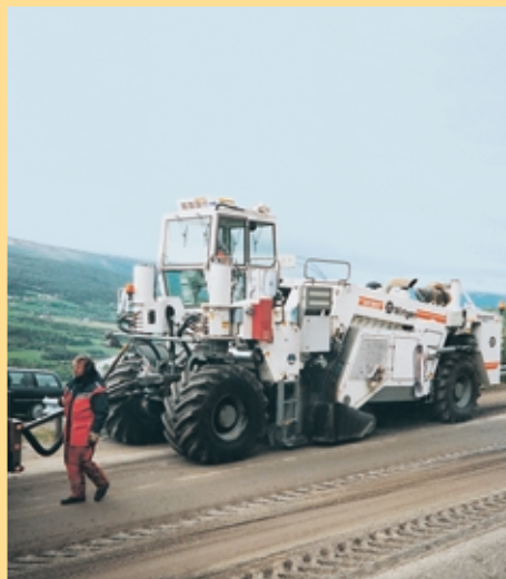
WR 2500 recycling a carriageway construction with addition of foamed bitumen.
