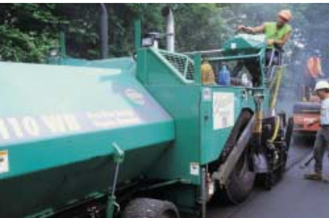
Superpave mix is placed in suburban Pittsburgh
