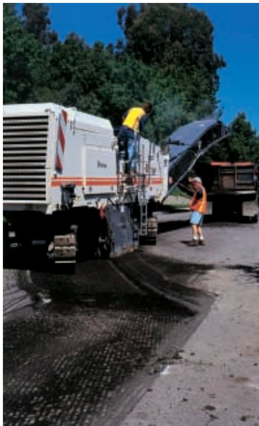
W 1200 mills laterally up local street
