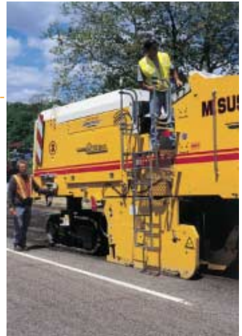
Susi's new W 2100 cuts Martin Luther King Blvd. in Boston's Roxbury neighborhood
