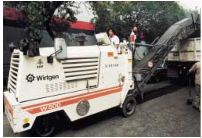
Cuauhtemoc public works' new W 500 at work
