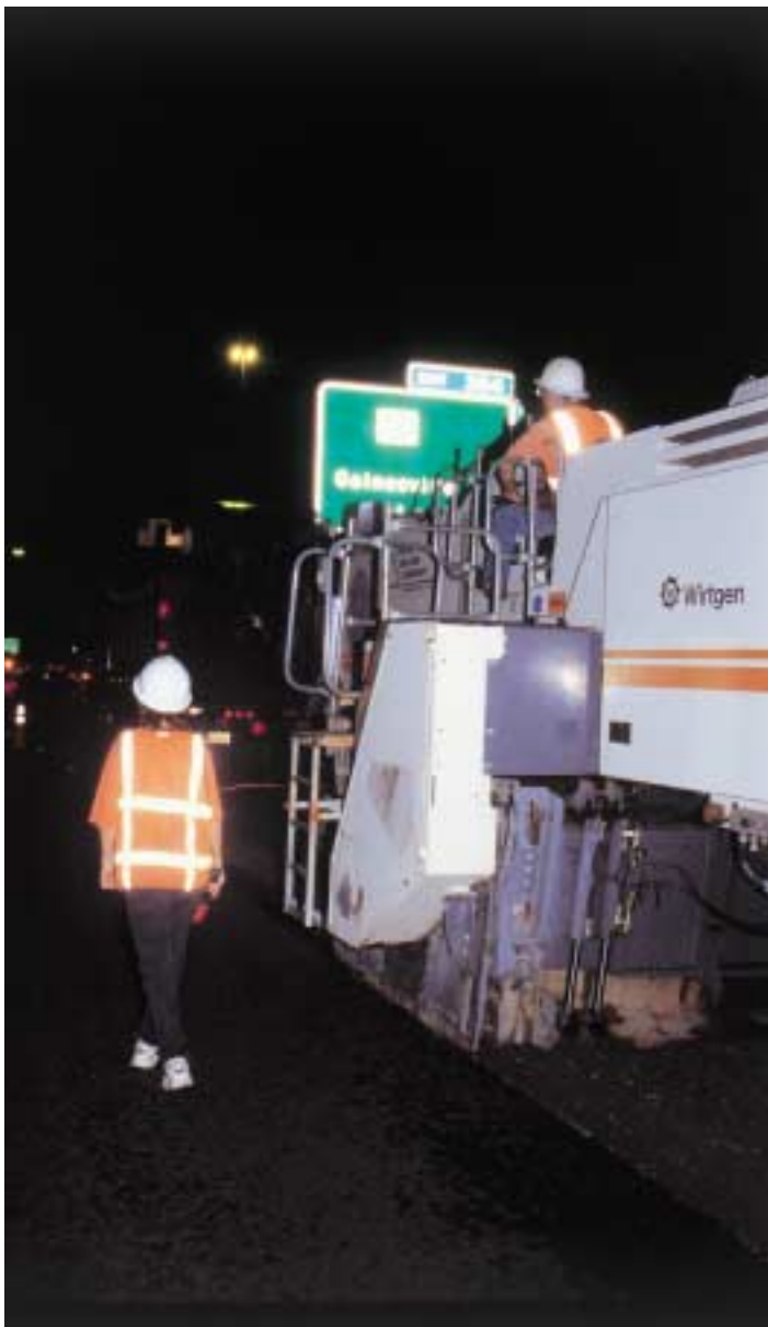
Milling at Gainesville exit takes place at night
