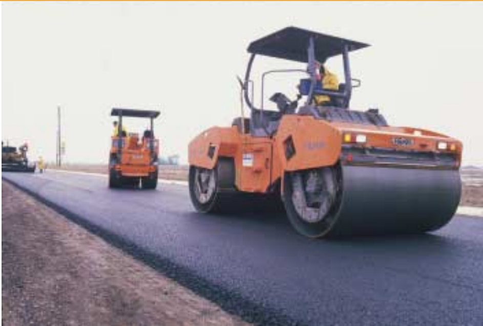
HW 90, HD 130 get quick compaction of mat
