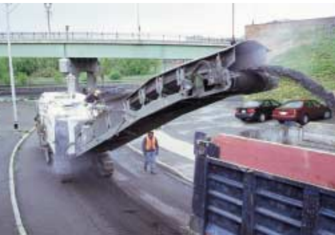
New York State DOT improves Amsterdam interchange
