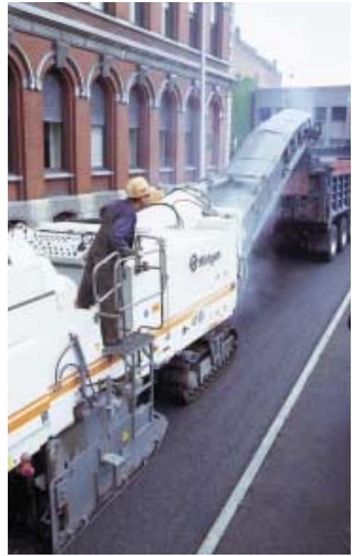
2100 DC handles tight quarters in Old Amsterdam, N. Y.
