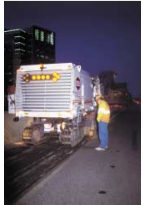
I-95 work in Stamford, Conn. begins at dusk
