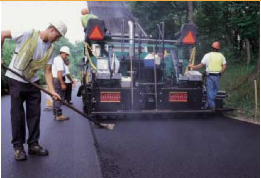
Vibration at screed makes Superpave placement easier
